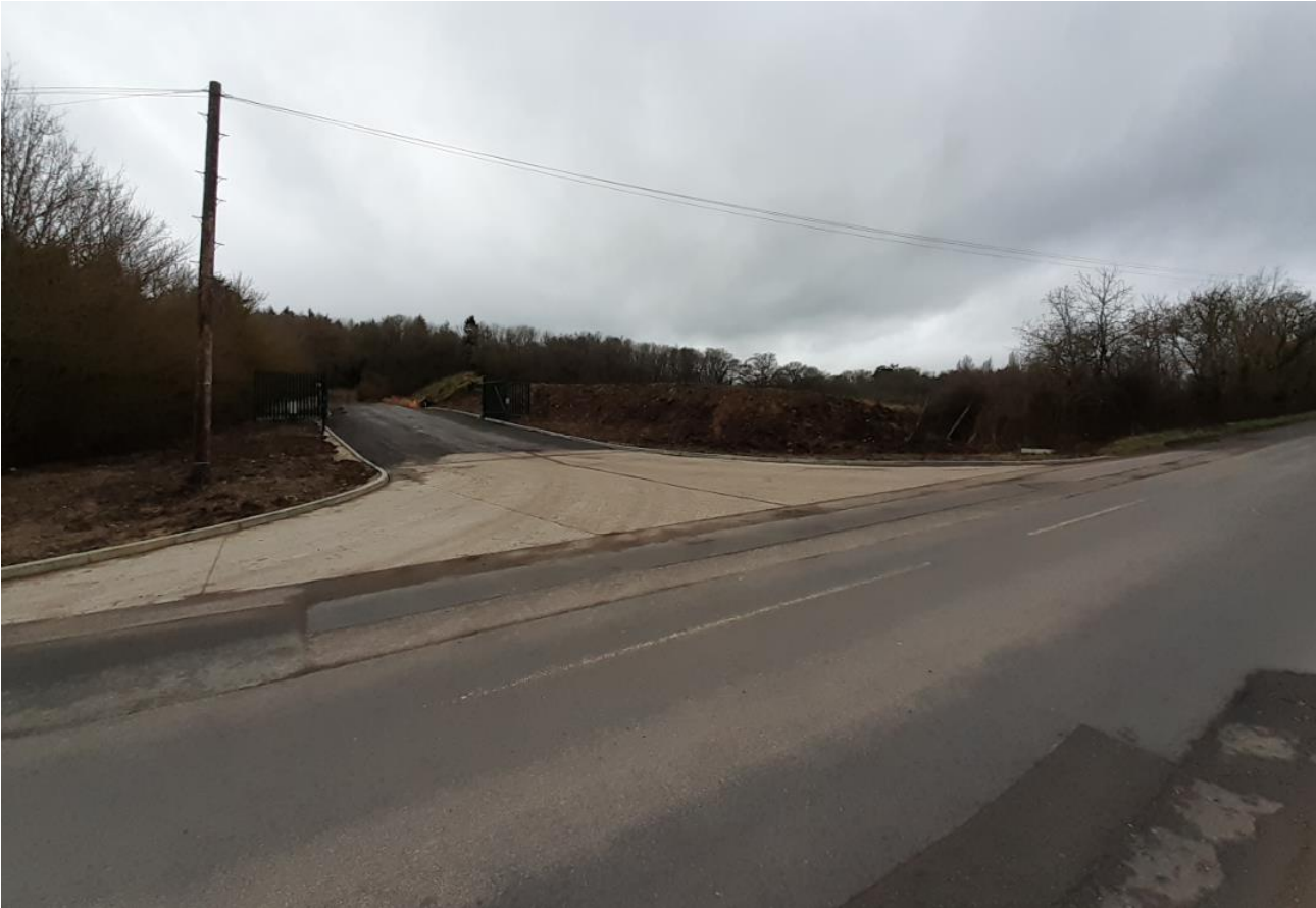
Figure 3 - View of partly completed bund from Bowling Alley
